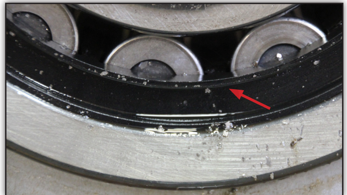
Metal flakes have pooled at the bottom of this bearing. It needs to be replaced.
